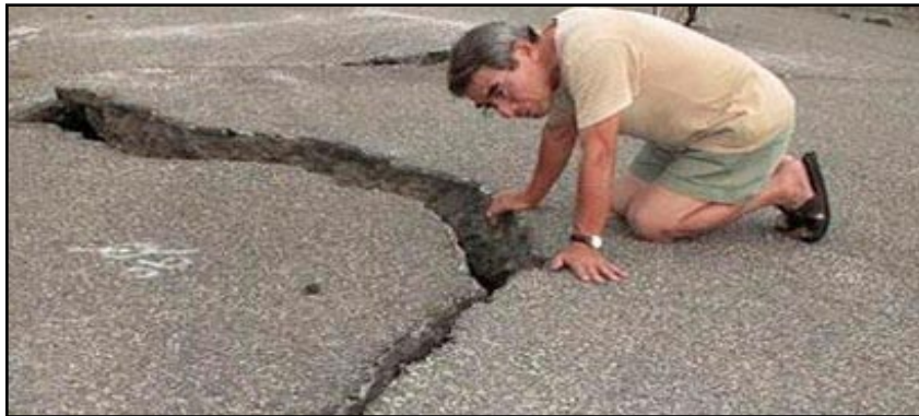
One man examines a large crack after the 9.0 earthquake in Japan Friday March 11. Photo from Justsharthis.com
